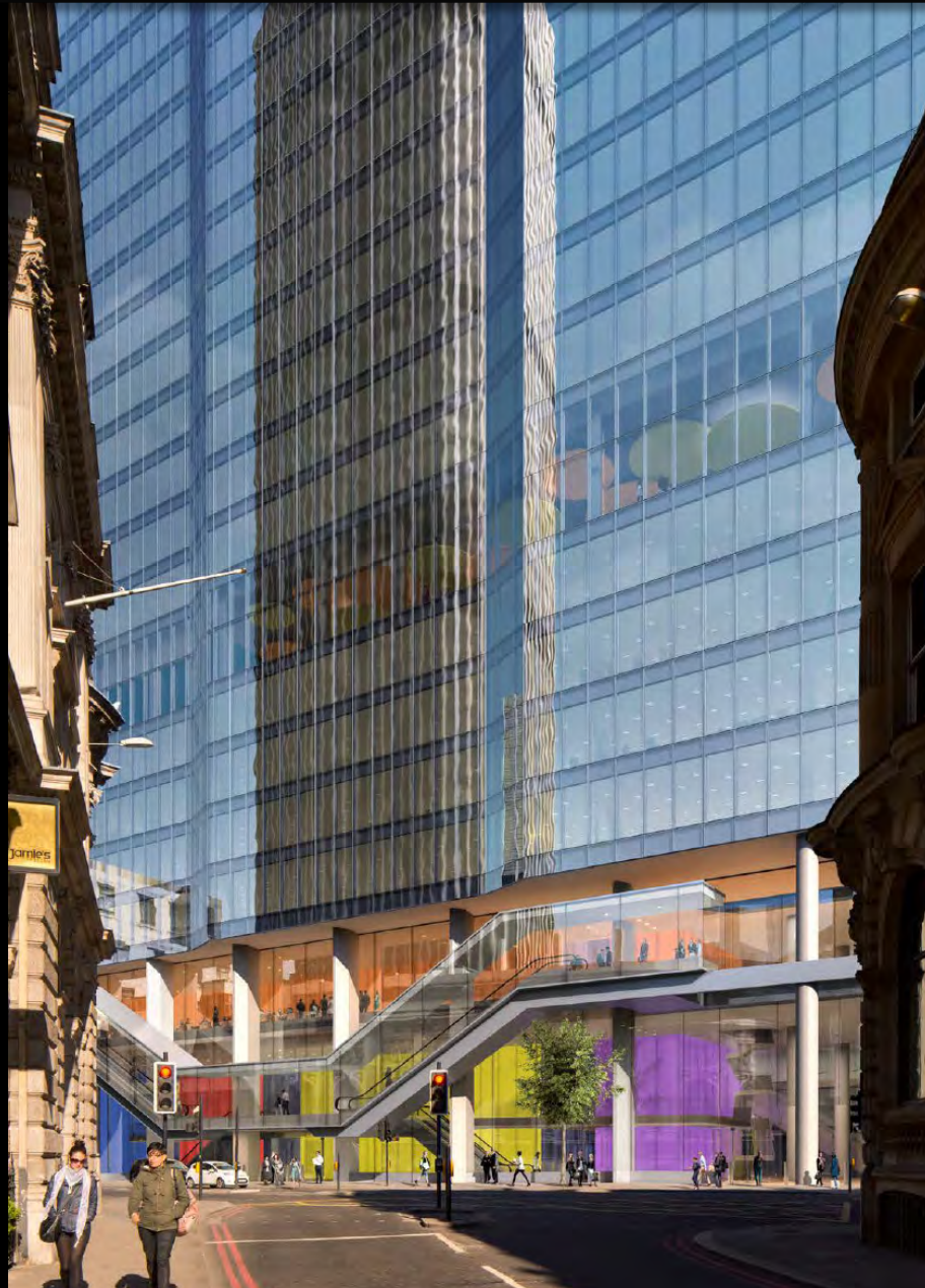
Bishopsgate frontage with Office lobby
