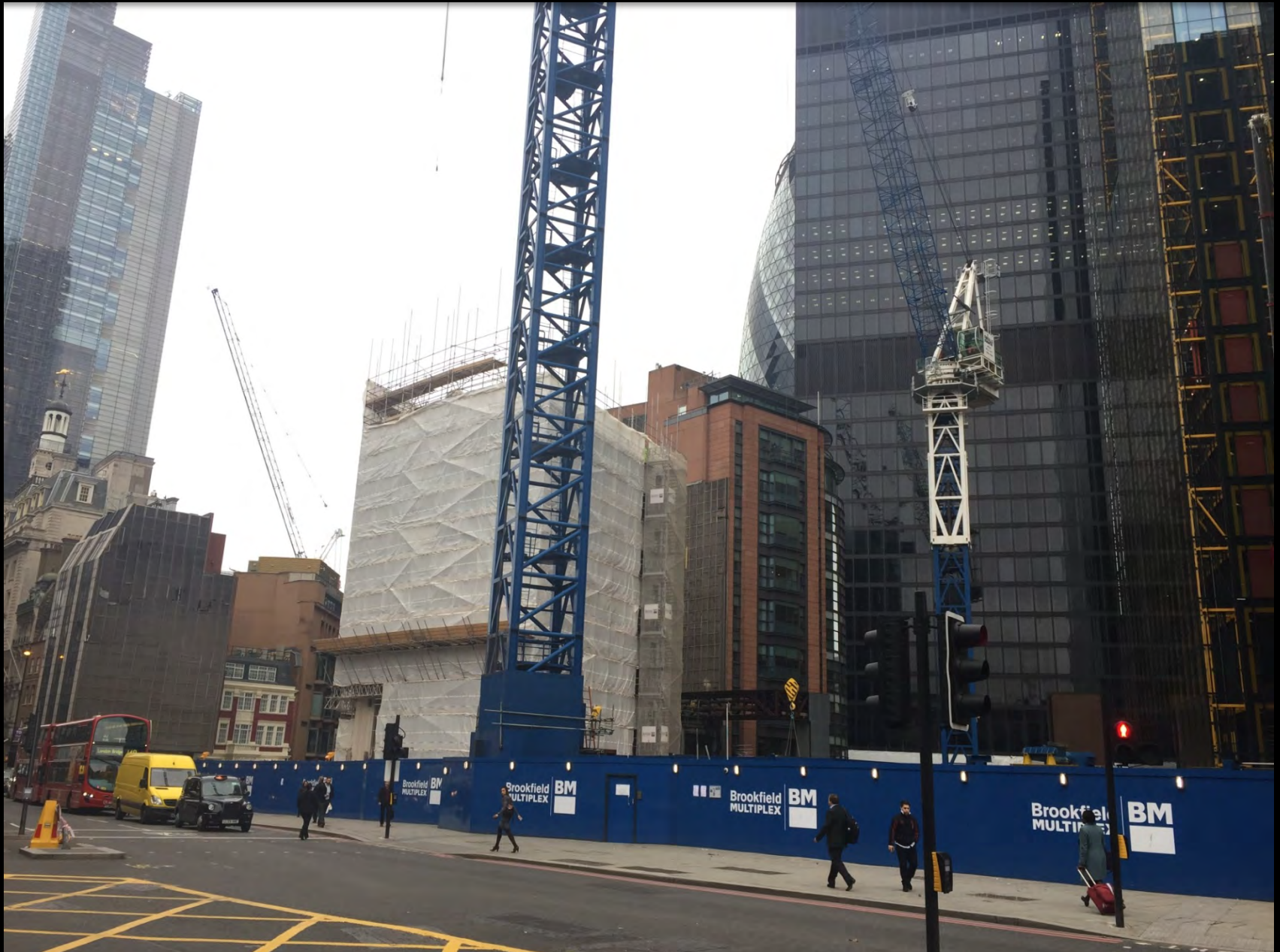
22 Bishopsgate construction site
